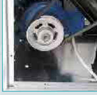
Belt drive and motor position.
